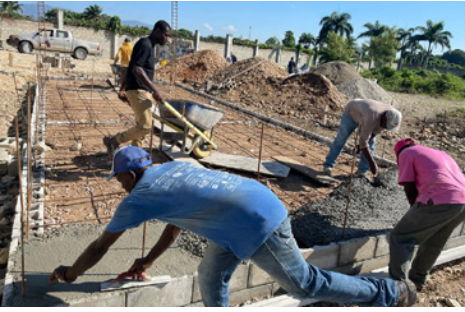
Starting work on the Caretaker's house, Espwa.
