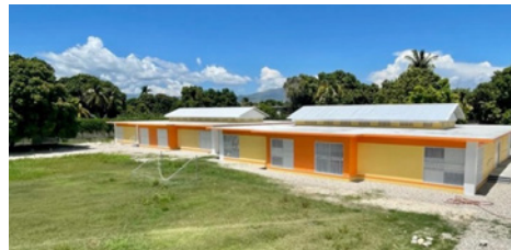
A view of the 4th classroom building and kitchen facility at Baryè Fè.
