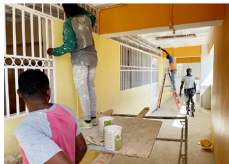
Maintenance work at Repatriote building 1 & 2.
