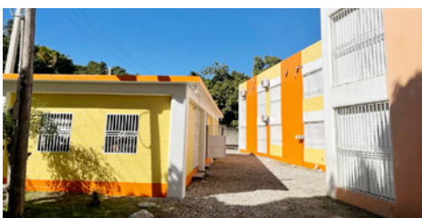
Picture of newly painted building 1, building 2 in right foreground and newly painted generator/toilet building in left foreground.
