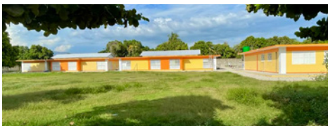
Baryè Fè, from left classroom building 3 (10th & 11th grade) classroom 4 (12th & 13th grade) and kitchen.
