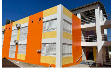
Building 1 painted, awaiting returning students.
