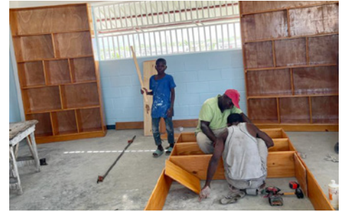
Installing library shelves in Youth Building.
